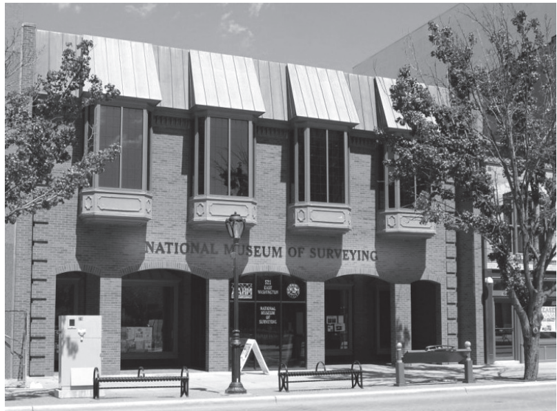
Located on E. Washington Street in Springfield, Illinois, the National Museum of Surveying sits between the historic Old State Capitol Building and the Abraham Lincoln Presidential Museum.
