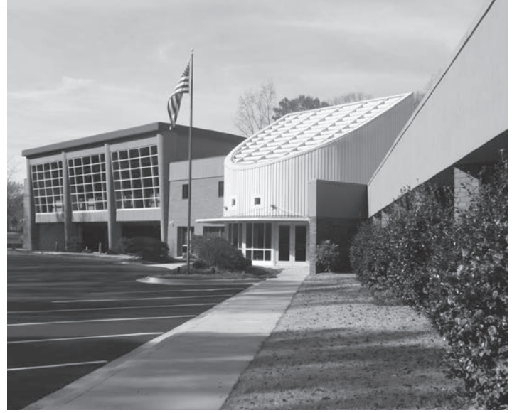
NCEES headquarters in Clemson, South Carolina, has a staff of 73 who oversee the day-to-day operation of the organization.
