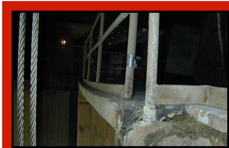
Large deflections easily visible
