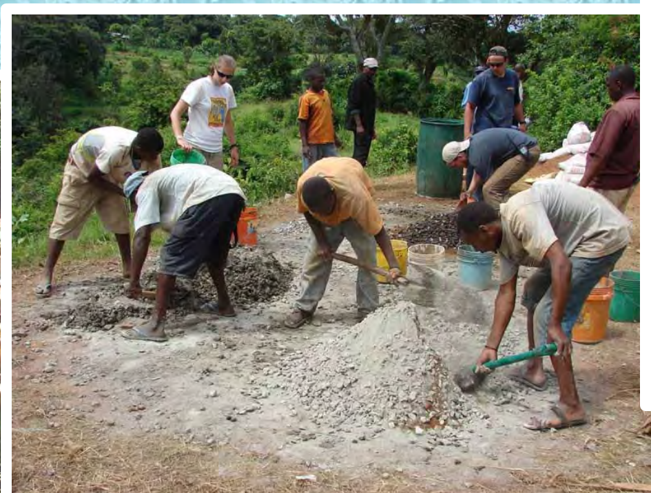
Training villagers in formwork (left), concrete mixing (middle), and concrete placement (top right), sample instructions for maintenance manual (bottom right).
