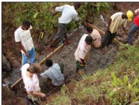
Figure 4: Villagers and EWB students tie the rebar for the drop box.
