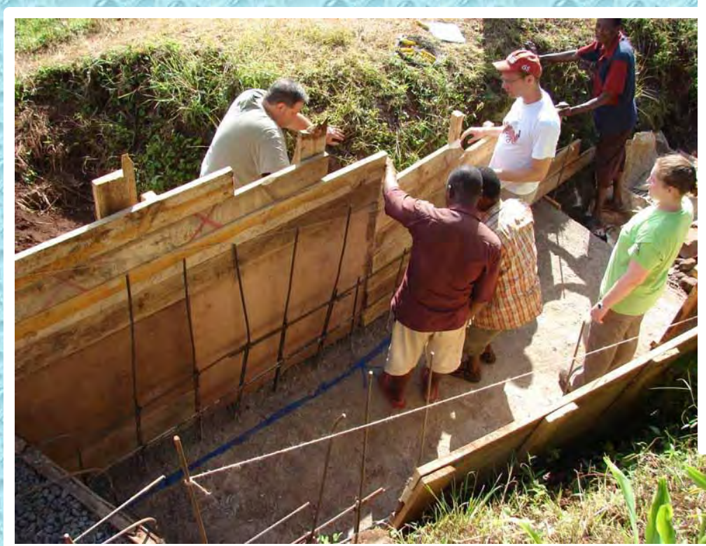
Training villagers in formwork (left), concrete mixing (middle), and concrete placement (top right), sample instructions for maintenance manual (bottom right).
