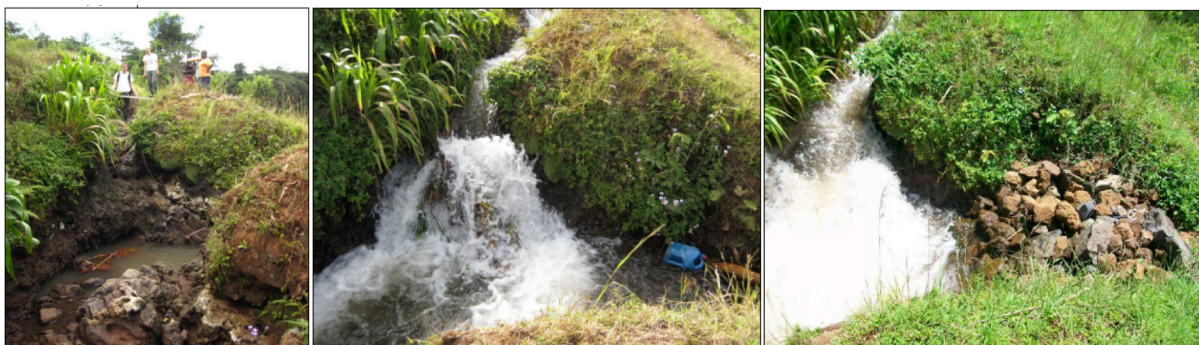
Figure 2: Junction 1 dry showing canal bed erosion (left), then with water flow showing runoff to the right (middle), and with emergency fix (rocks) implemented in 2010 (right).
