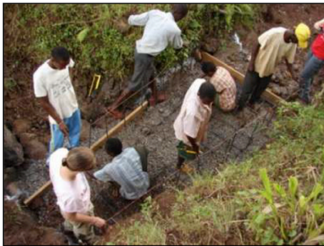
Figure 4: Villagers and EWB students tie the rebar for the drop box.
