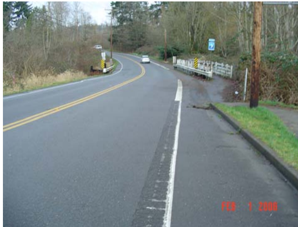
Figure 1. Bridge alignment (looking south)
