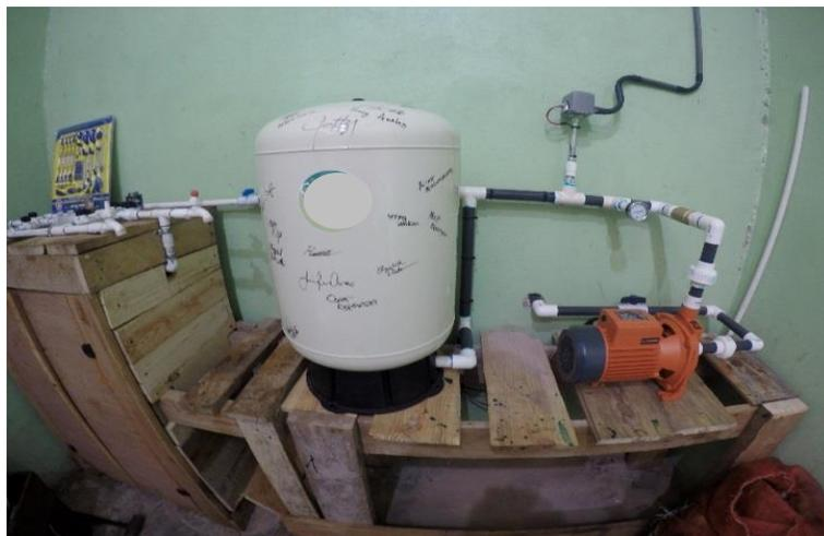
The water is initially pumped from the existing well to the 300 gallon storage tank which sits atop the 13 foot concrete tank base. The storage tank is then gravity fed to a 1 hp pump that begins to fill up the bladder tank which directly supplies pressure to the kitchen faucets. The water being pumped to the kitchen goes through a 0.5 micron filter before
