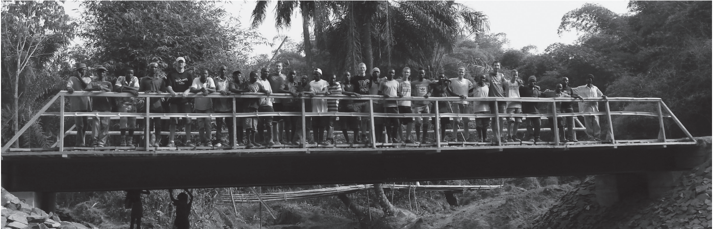
Participants with the Dordt College Engineering Department celebrate the completion of their Liberia Farm bridge. The project, which won the $25,000 NCEES Engineering Education Award grand prize, took students and practitioners from designing a bridge in Sioux Center, Iowa, to building it in Monrovia, Liberia.
