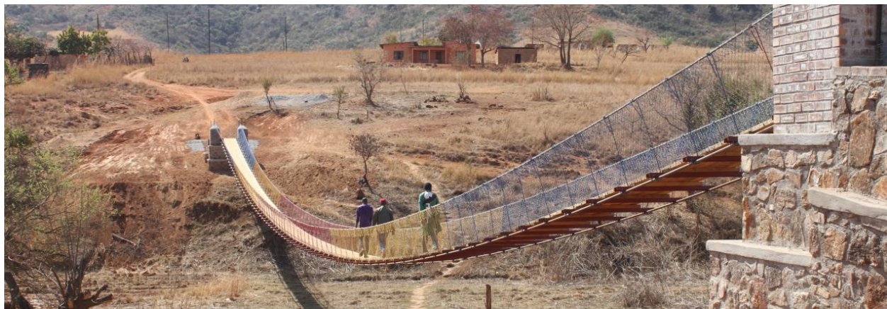
Figure 8. Final Constructed Bridge
