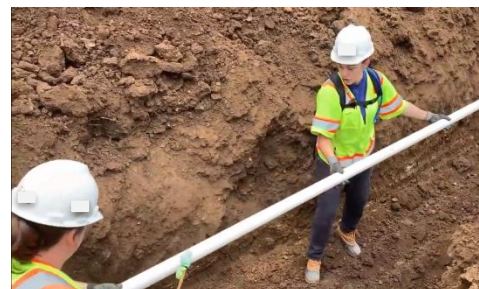
Figure 3: Installation of Distribution Piping
