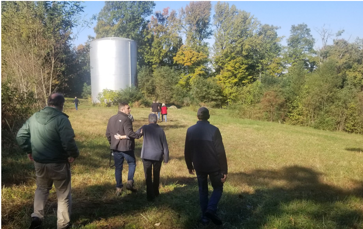
Figure 1: Existing Water Tank
