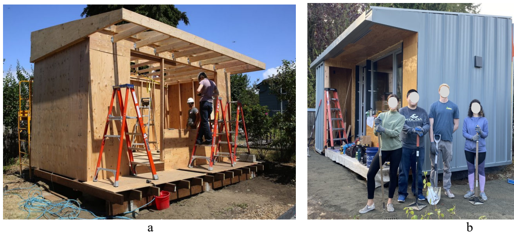
Figure 1. Accessory Dwelling Unit a) under construction, b) Student volunteers at work
