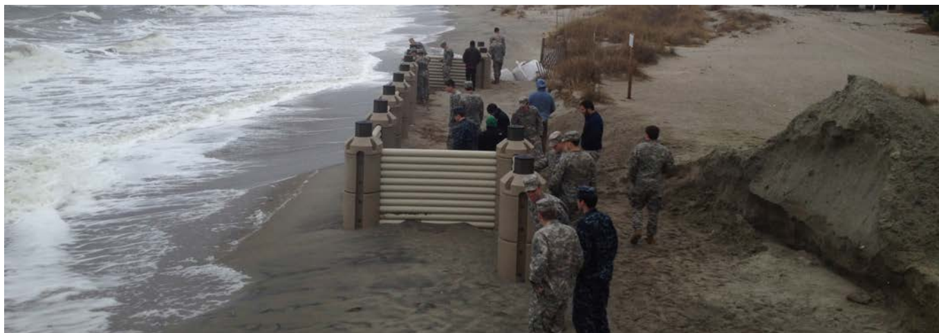
Figure 8. University A research team performing an assessment of the Wave Dissipation System following a storm event.
