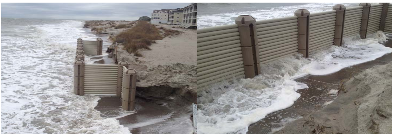
Figure 5. Installation of prototype Wave Dissipation System.
