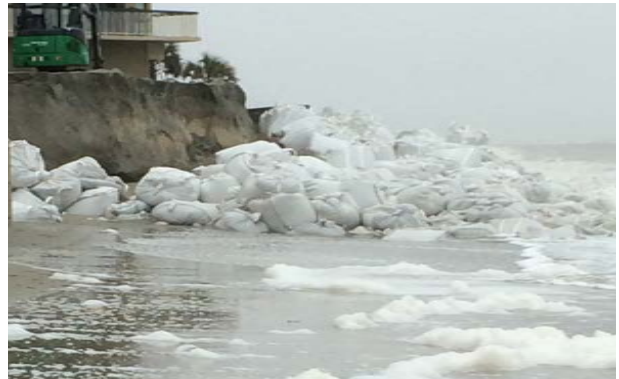
Figure 2. Typical sandbag installation following a storm event.
