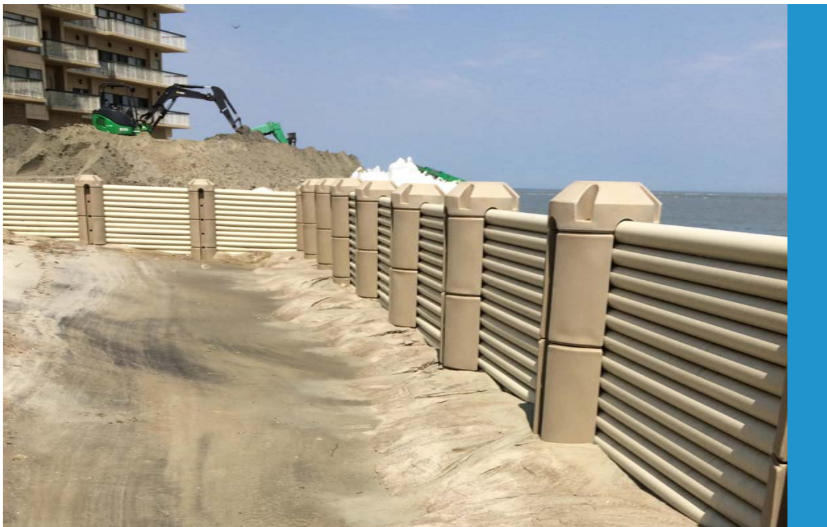
Figure 7. Sand accretion behind Wave Dissipation System following high tide.
