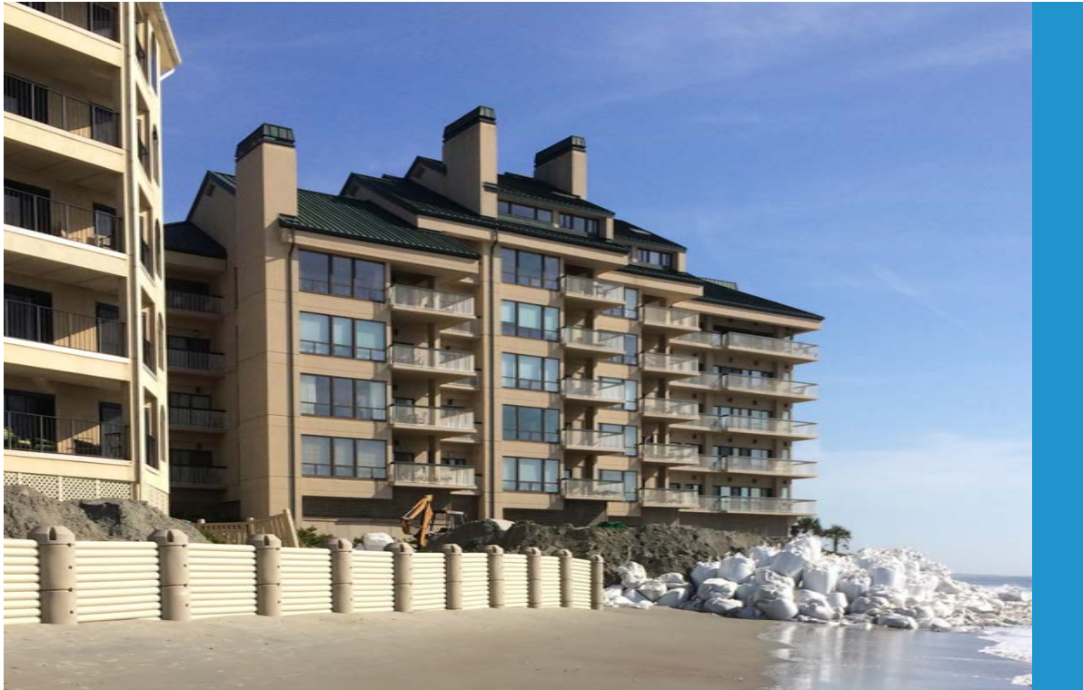
Figure 6. Installation of complete Wave Dissipation System for building protection as an alternative to sand bags. Aproximate cost was $500 per linear ft.
