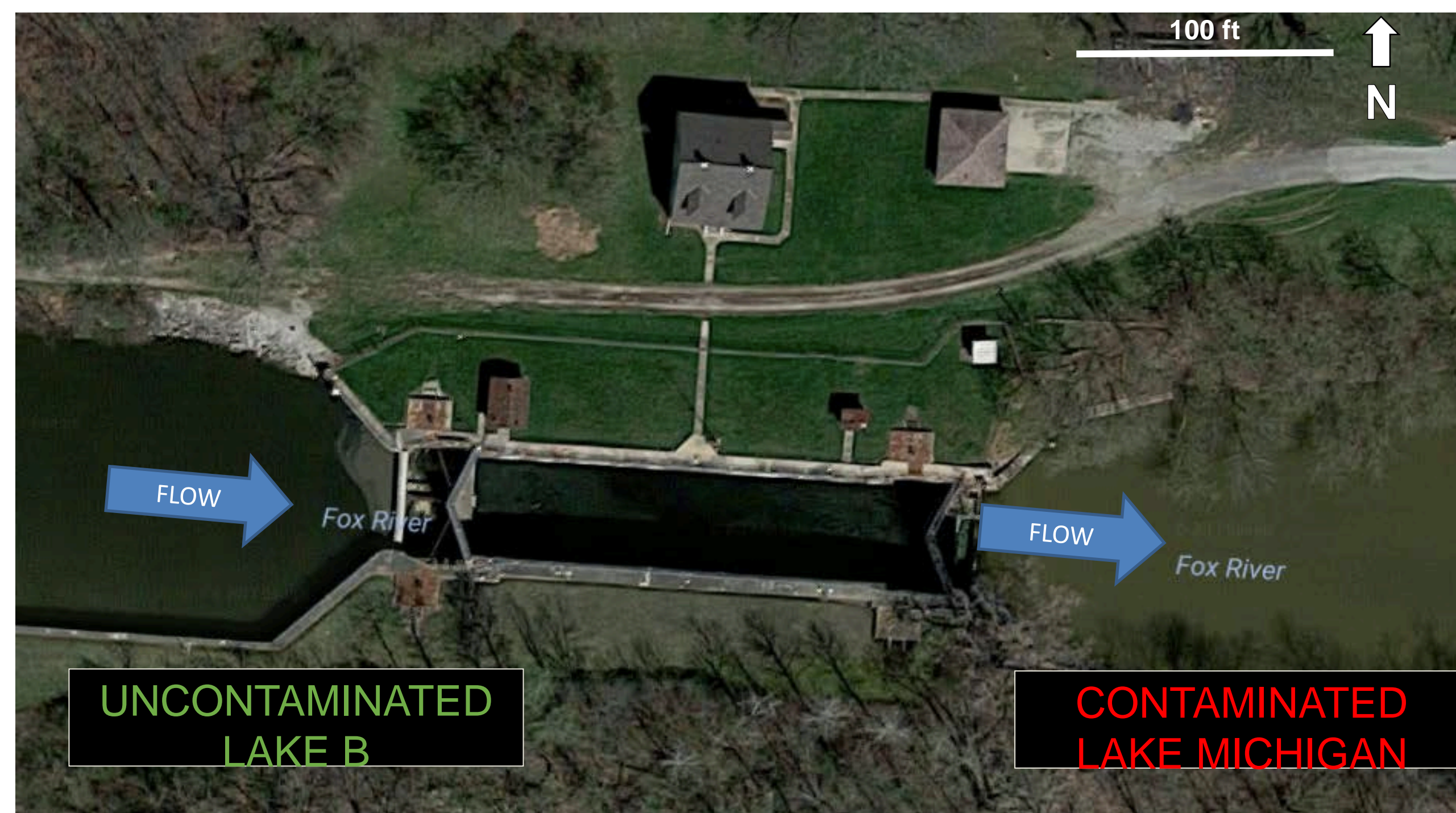
Figure 1. Interlake Lock and Boat Transfer
