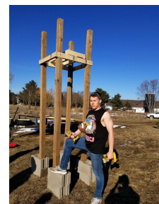
Figure 4: Team member assembling early tower prototype at a build day
