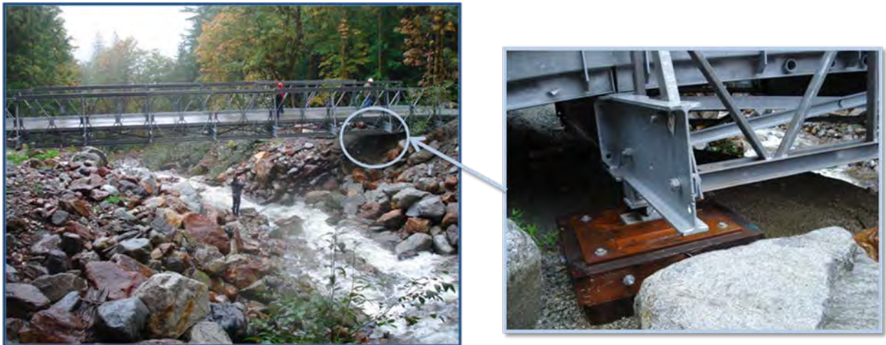
Figure 1. Modular Bridge on Temporary Timber Support
