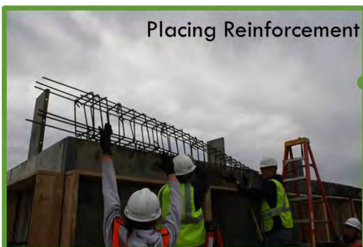
Reinforcement Preparation
