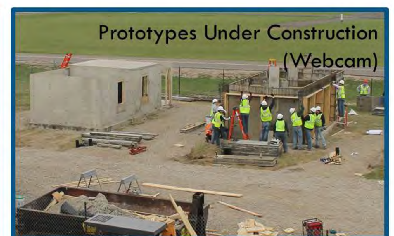
Formwork Erection
