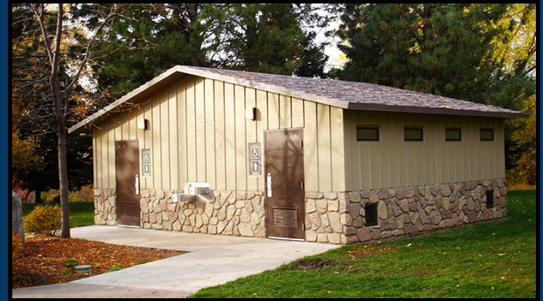
Fig. 32 Example of Park Restroom Structure.
