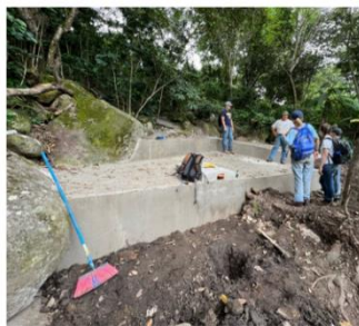
Completed spring box (left) and distribution tank (right)
