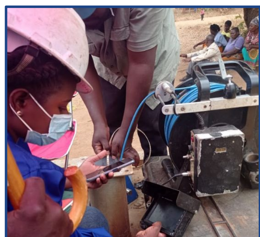
Camera survey of borehole
