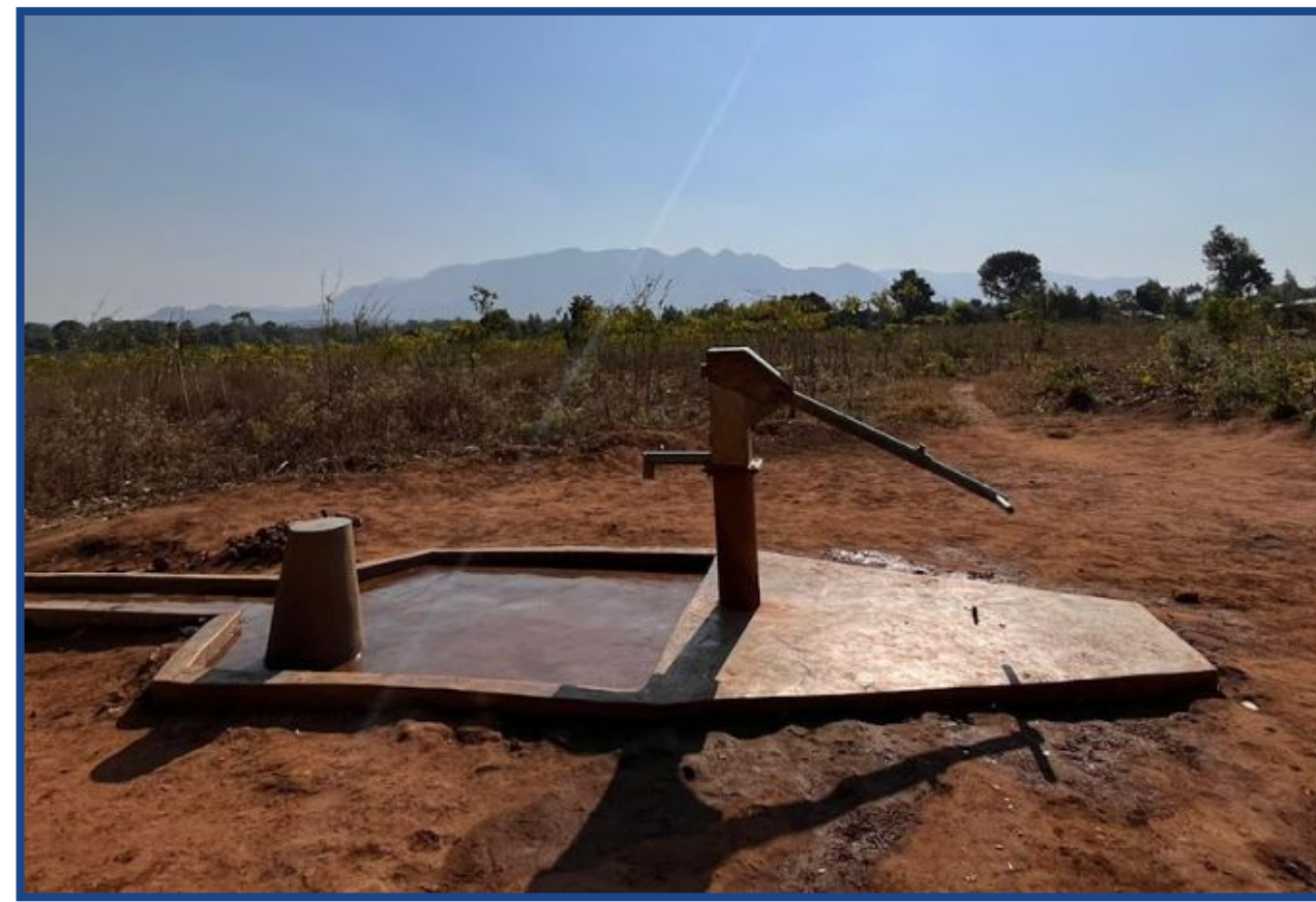
Borehole well in Malawi
