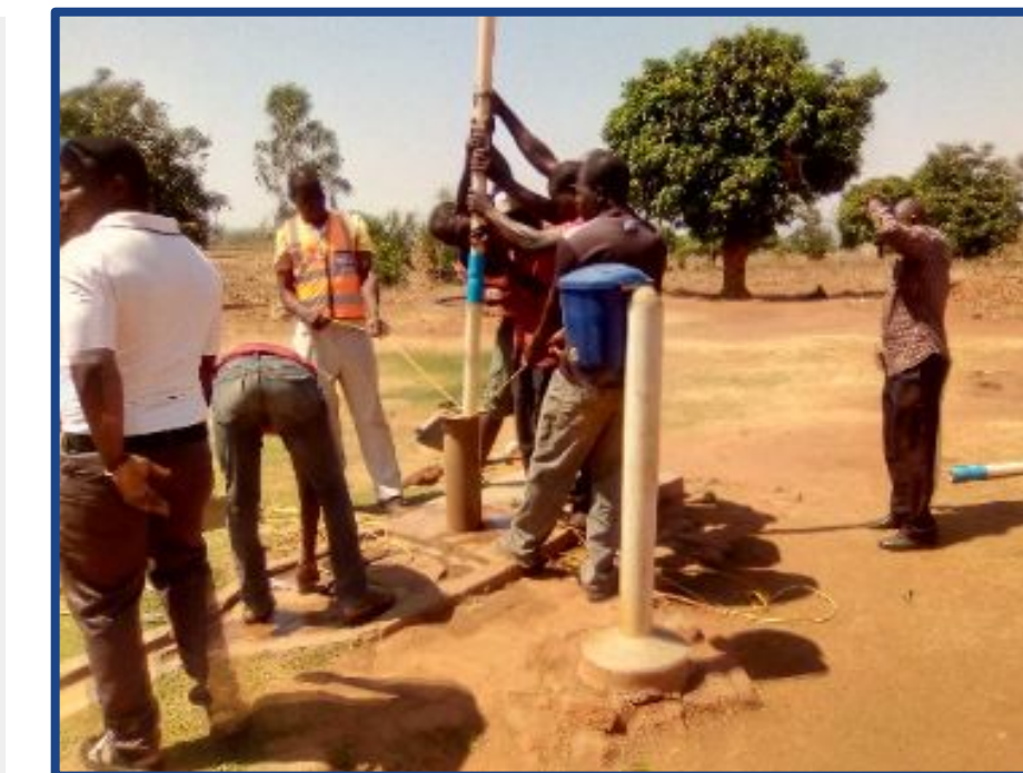
Replacing well parts in Nkagula
