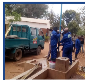
Inspecting well casing
