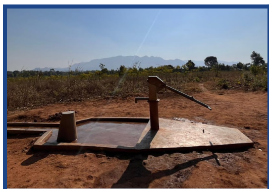
Borehole Well in Malawi
