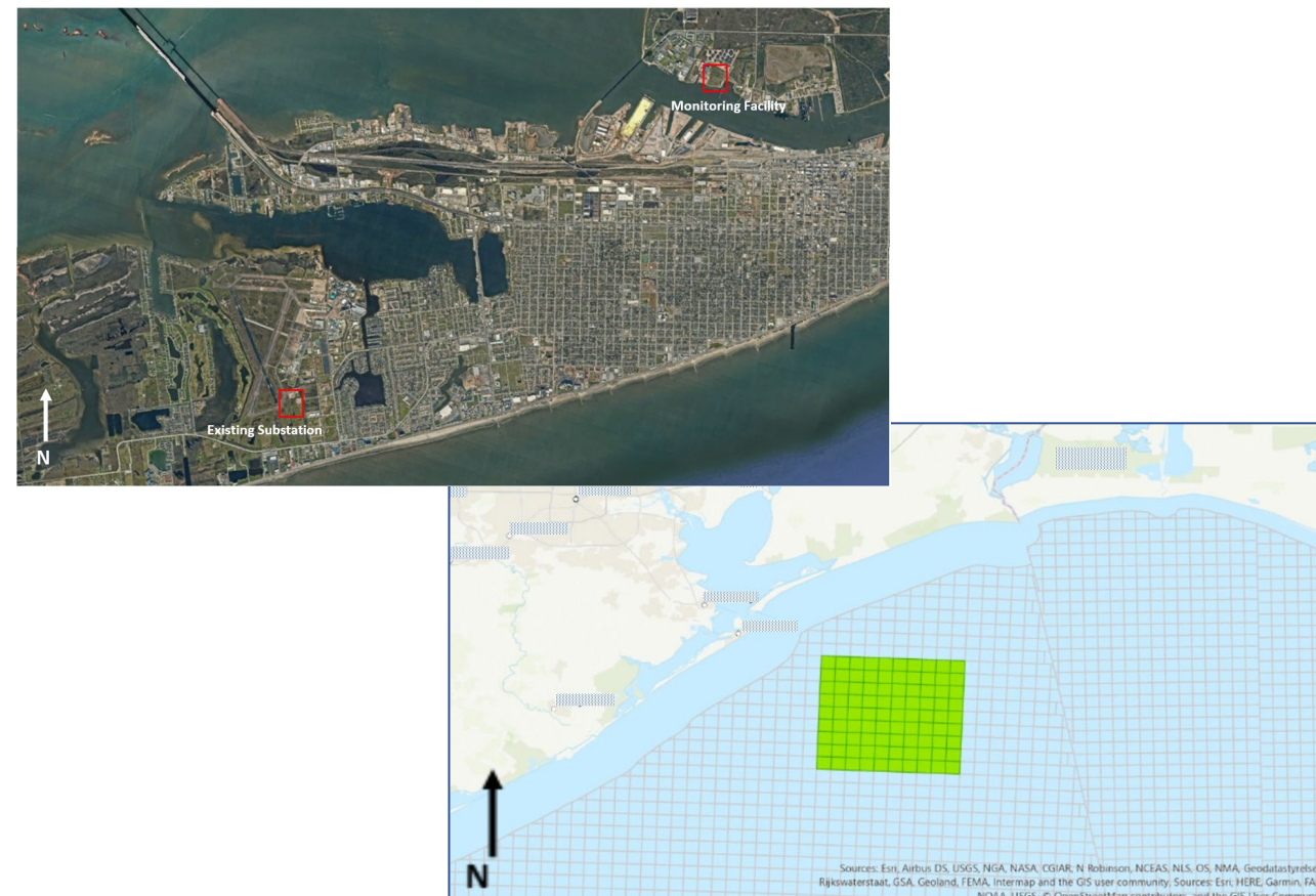
Existing Substation and Land Area (top right) and Wind Farm Lease Blocks (bottom left).
