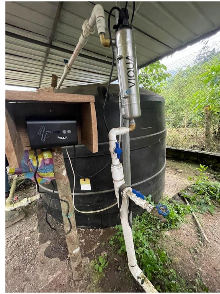
Ultraviolet Light Water Disinfection system able to clean up to 16 gallons / minute.
