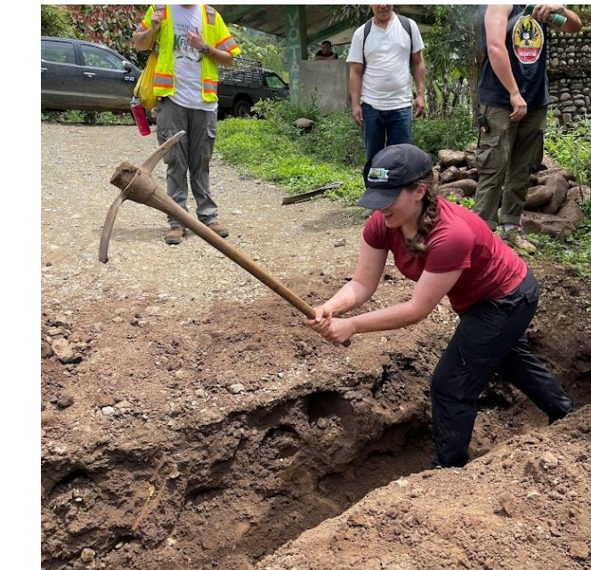
A student digging the trench for the installing the conduits.
