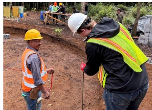
EWB-Guatemala Engineer teaches a student to level a surface with water.
