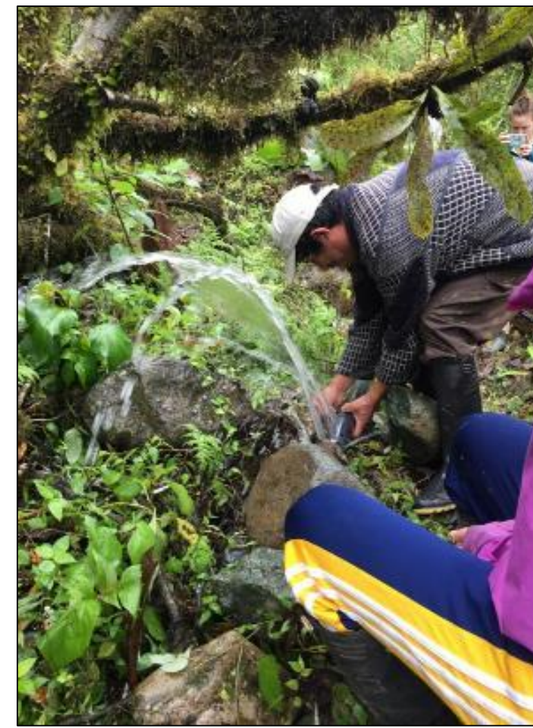
A Community Member fixing a leak in the existing water system.
