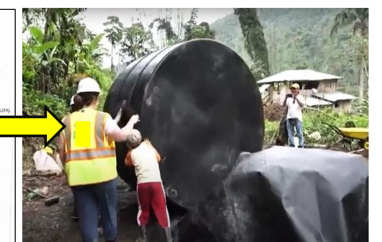
Water Storage Tank Construction
