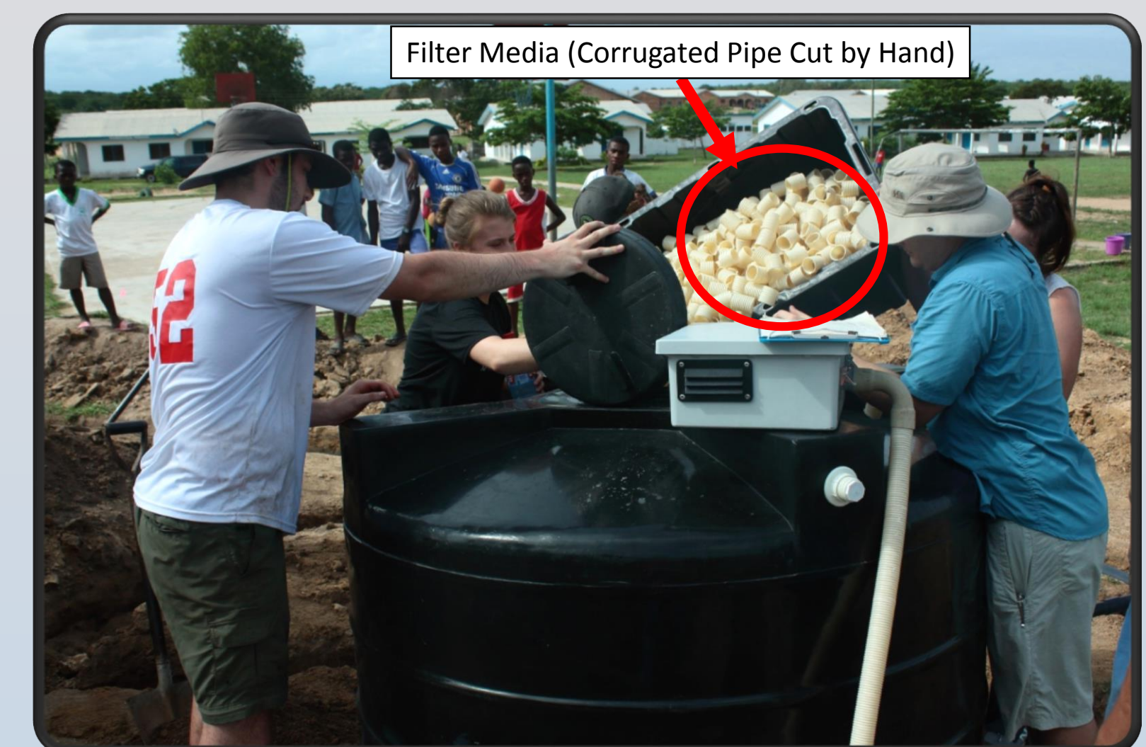
Figure 6: Filter media inserted into the filter tanks for treating the wastewater
