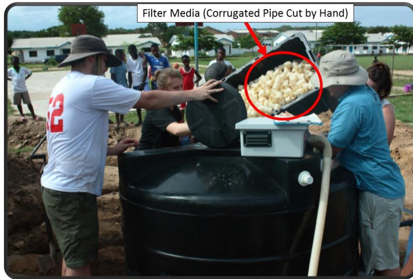
Figure 5: Approximately 30 tubs of filter media cut by hand was added to the two filter tanks
