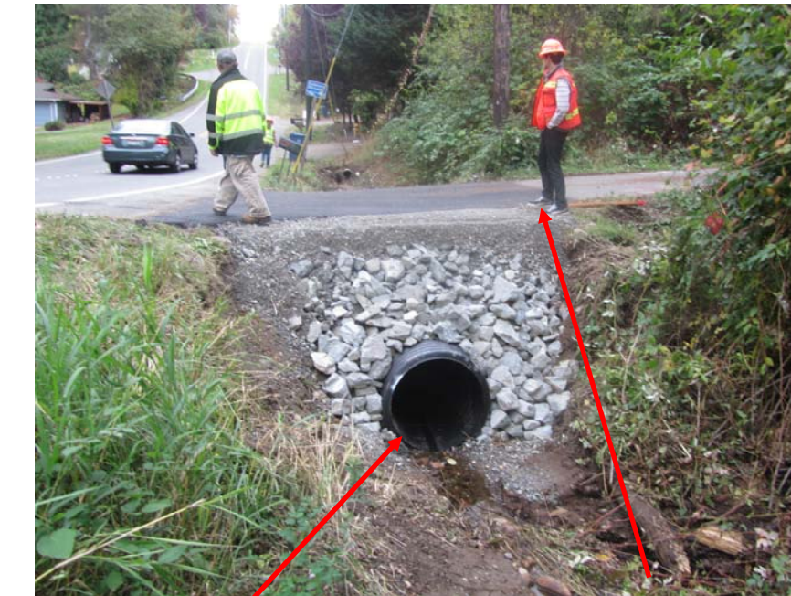
Driveway culvert Team member at work
