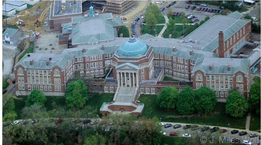
Figure 2: Existing high school at East side of site
